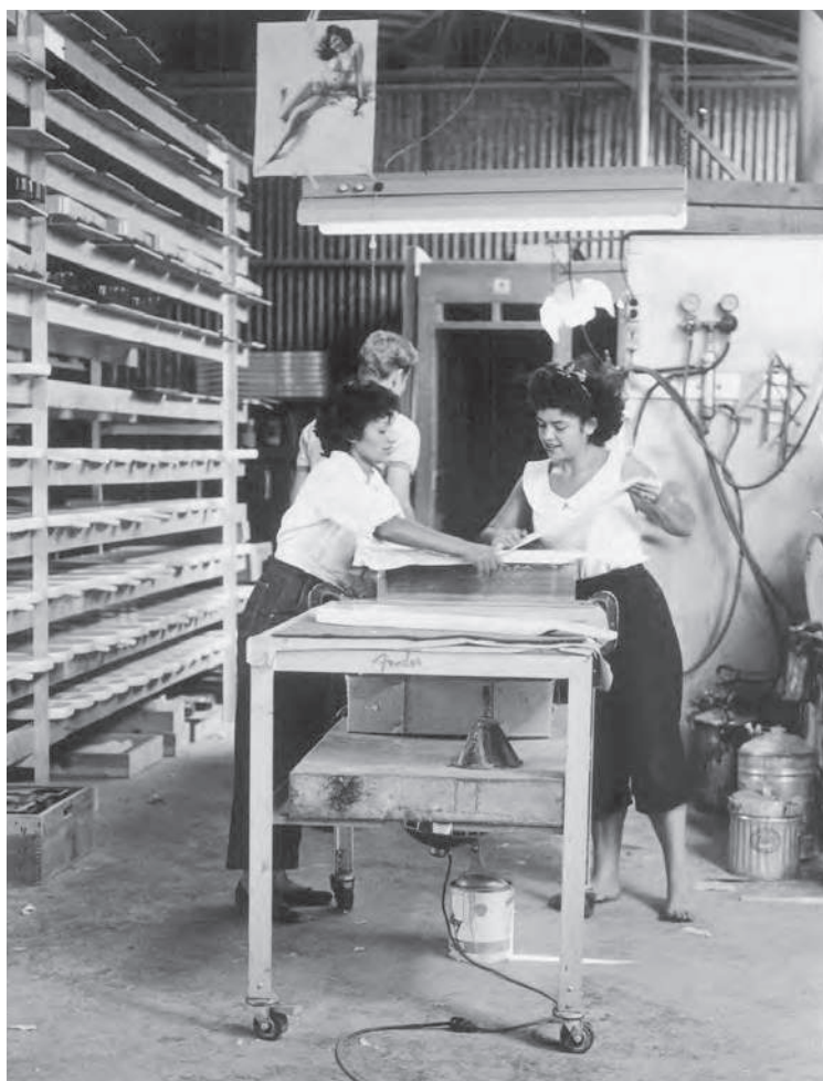
Irene Vasquez (left) and a colleague cover a Fender lap-steel in acetate.
